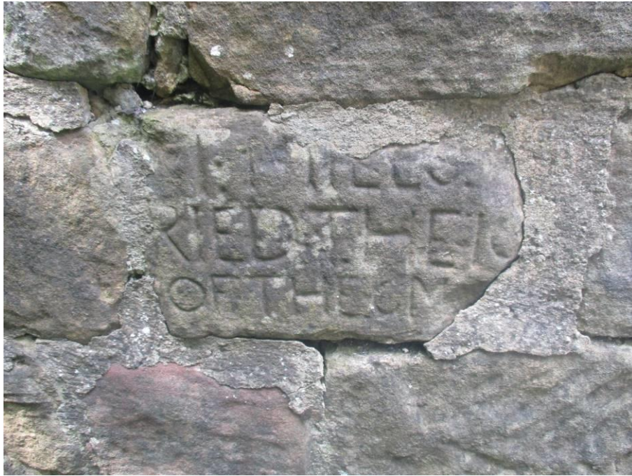
Figure 6: Example of re-used headstones in boundary wall
